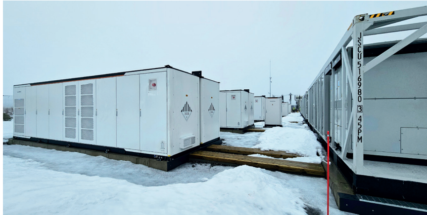
PowerTitan 1.0 and the corresponding PCS/MVS containers are installed close together.
