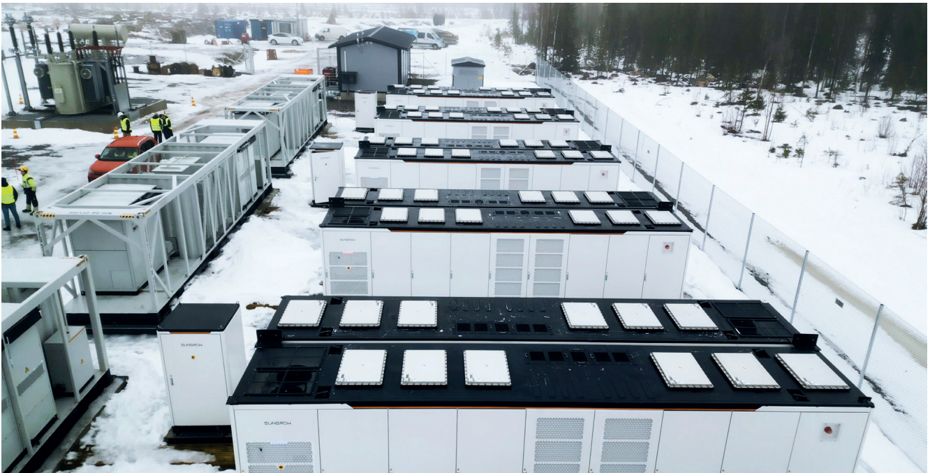
PowerTitan 1.0 can be installed back-to-back with no loss of performance.
