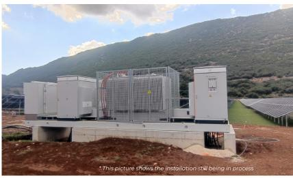
Two Sungrow SG3125HV-30 inverters are intalled in a skid solution with transformer and switchgear.
